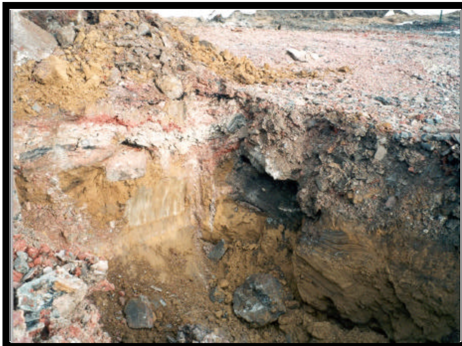
FIGURE 20. Excavation showing friable asbestos waste (red, white & black) and plate scrap.
