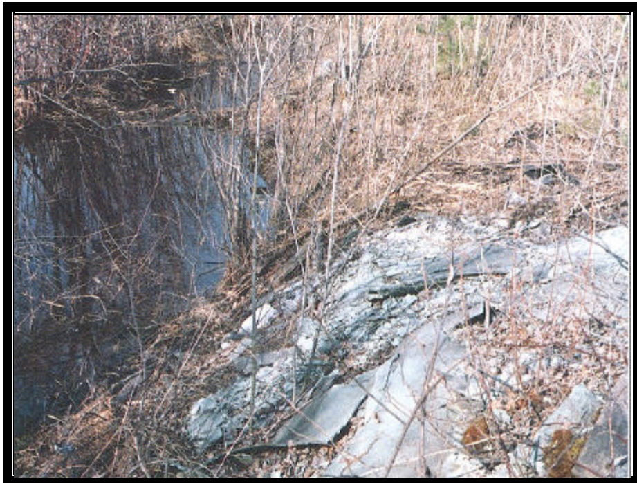
FIGURE 12. Piles of gray or colored sheets on the ground, or found buried in the ground.
