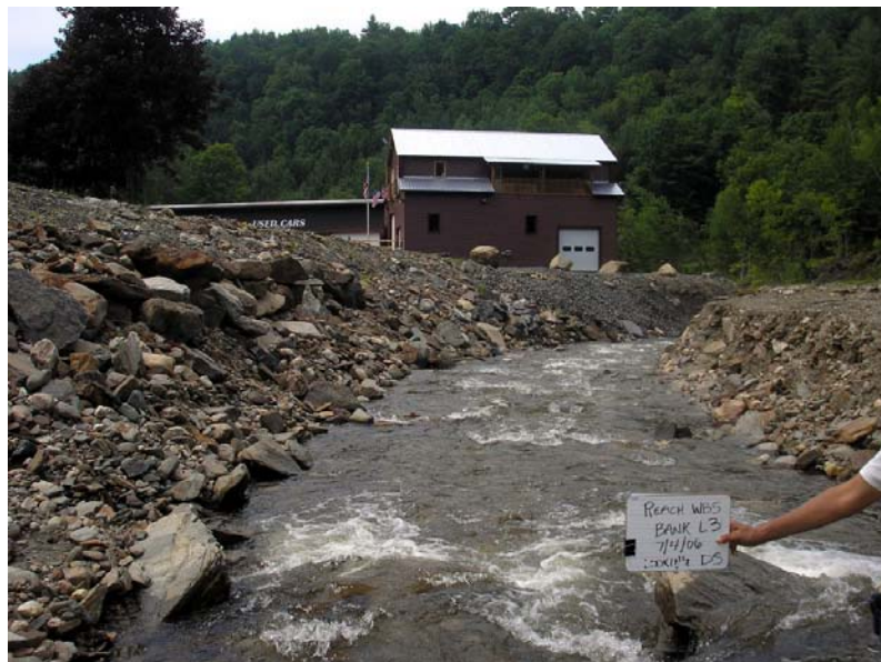
Figure 6-14: Photograph of channel degradation and widening on Warren Brook in Alstead, NH (Source: Horizons Engineering, LLC).
