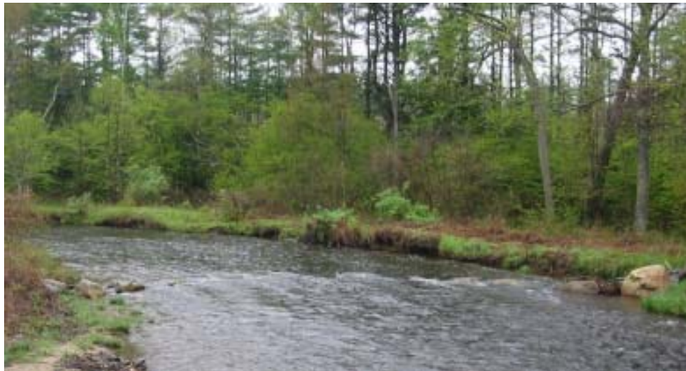
Figure 2-3: Photograph of a semi-natural form design on the Piscataquog River in New Boston, NH where a rock vortex weir (pictured above) and rock groins, or barbs, were used to limit erosion, protect infrastructure, and improve habitat (Source: MMI).
