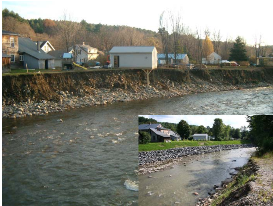
Figure 6-15: Photograph of an eroding bank associated with channel degradation on Warren Brook in Alstead, NH (Source: Horizons Engineering, LLC). Inset photograph shows the same bank following stabilization with riprap and grass.
