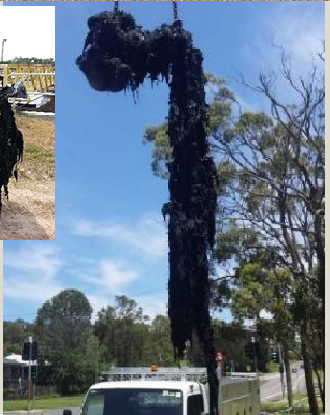
Eleebana Sewer Monster, Australia
