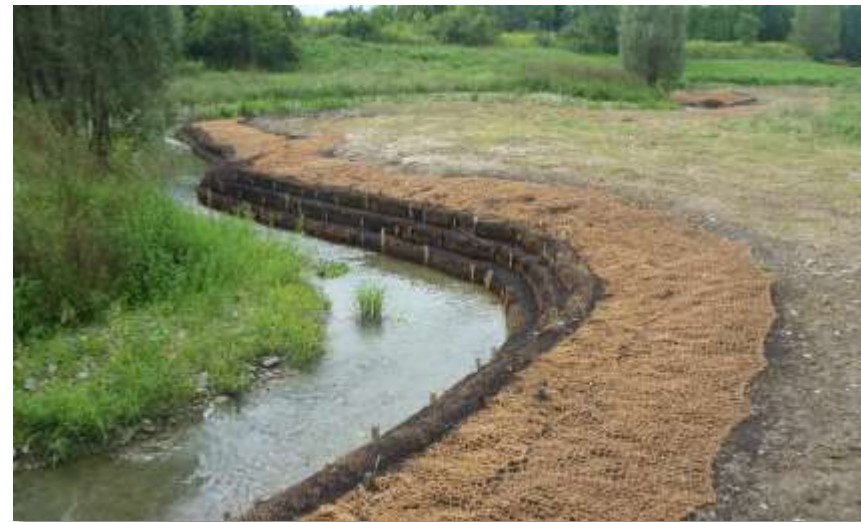
Wood additions create pool habitat for Brook Trout in Nash Stream
