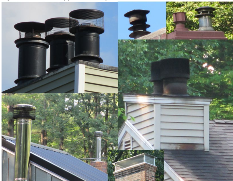
Figure 3.1: Metal Capped Chimneys
