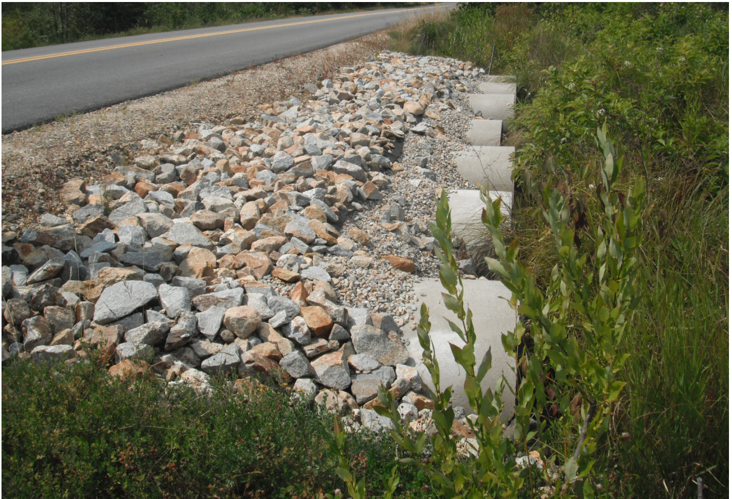
Coffin Brook restoration culverts, Alton, NH
