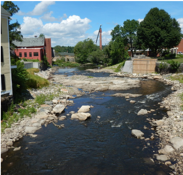
Great Dam removal and Exeter River restoration, Exeter, NH
