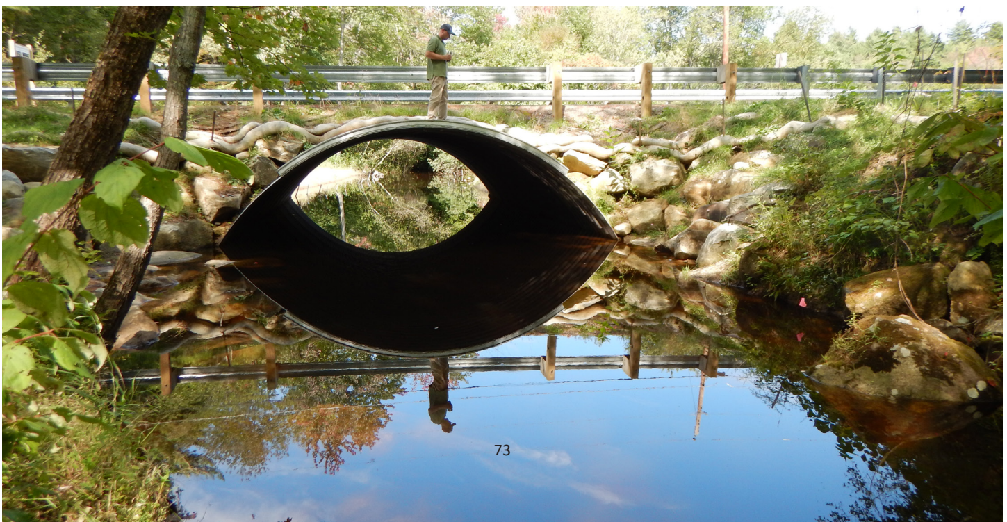
Falls Brook culvert replacement at Hale Hill Road, Swansey, NH
