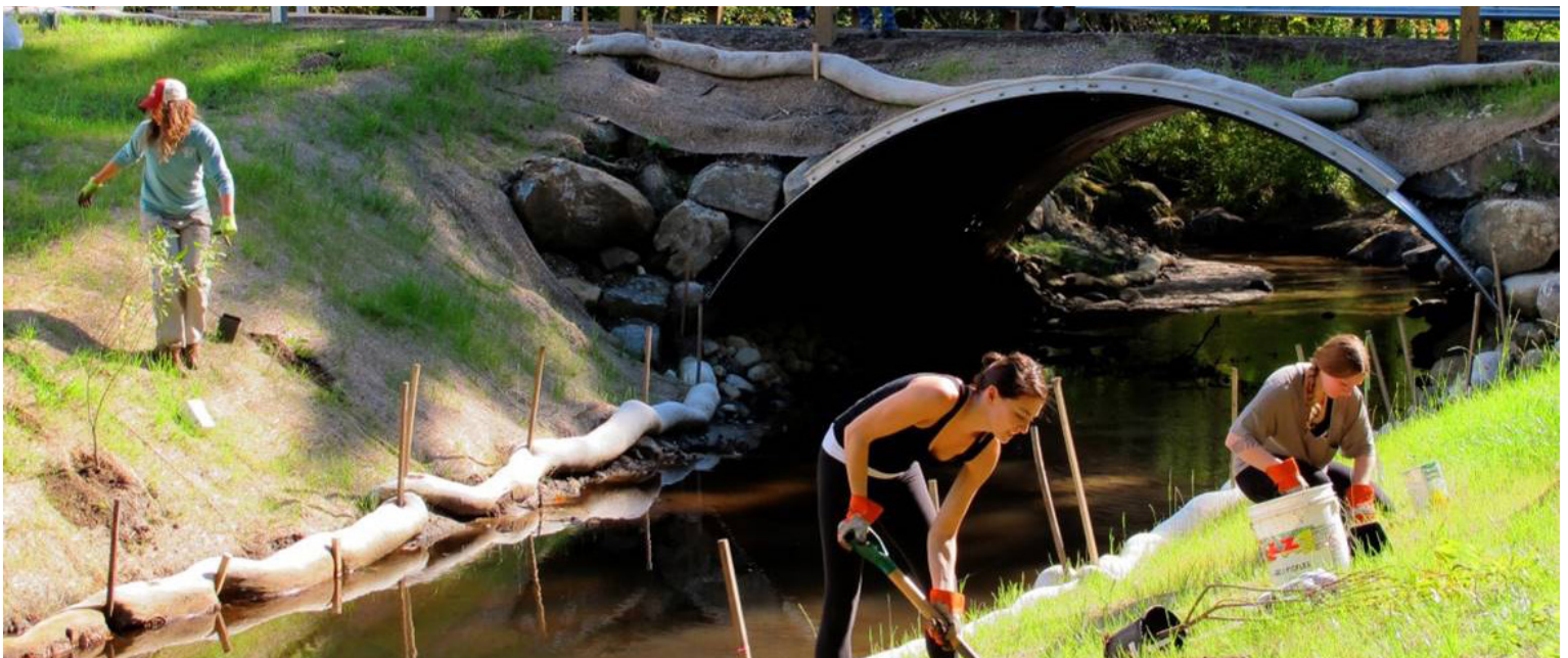
Falls Brook culvert restoration project – Lower Connecticut River watershed
