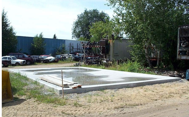
Concrete crusher pad under construction at local yard.
