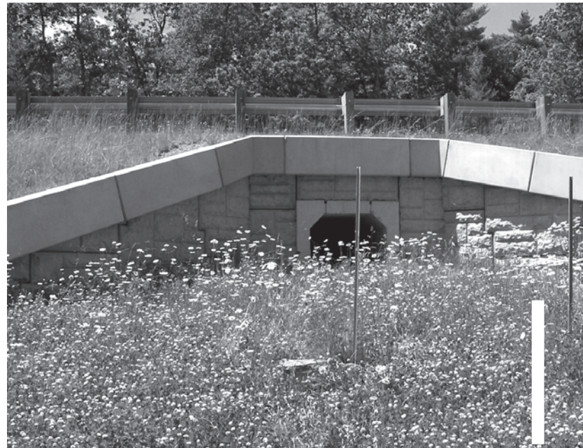
This tunnel in Windham, N.H., was created specifically for wood frogs and spotted salamanders.
