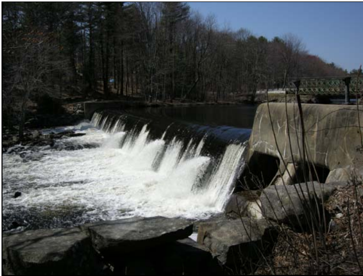
Figure 1 – Wiswall Dam, photo taken April 19, 2008.
