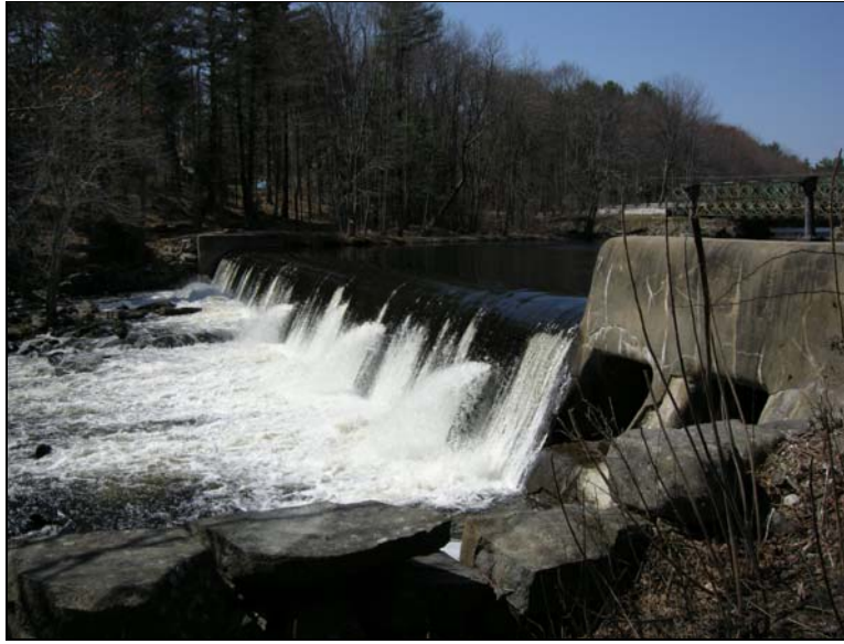
Figure 1 – Wiswall Dam, photo taken April 19, 2008.
