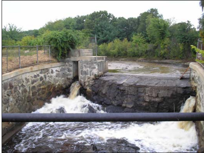
Figure 1: Maxwell Pond Dam. (September 2008 photo)
